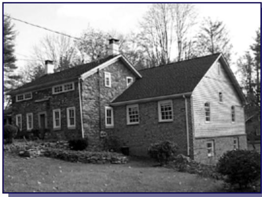
Figure 8. Front Elevation of Completed Project.
