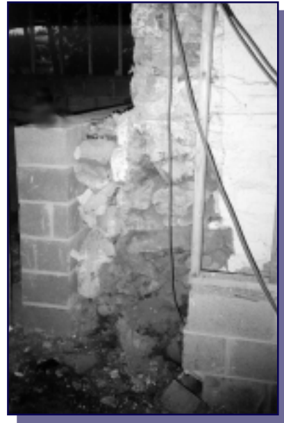
Figure 13. Rubble Stone Foundation.
