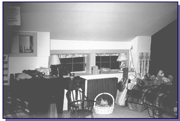
Figure 15. Existing 14- x 36- Inch Sliding Windows.
