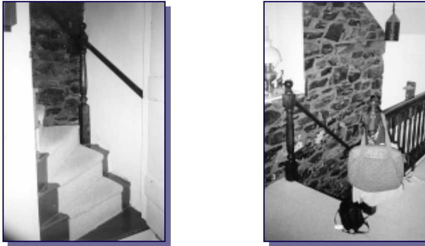
Figure 18. Existing Pocket Stairway.
