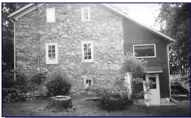
Figure 6. Carriage House and Porch.
